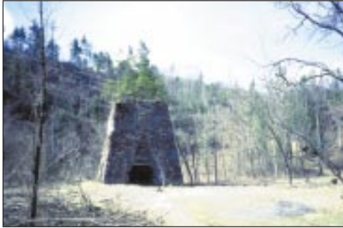
Old iron furnaces are common in some parts of western Virginia.
