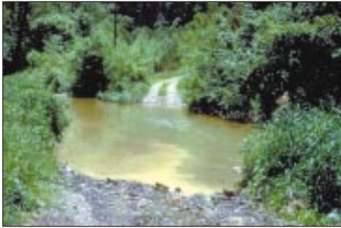
A ford can be an acceptable temporary stream crossing.
