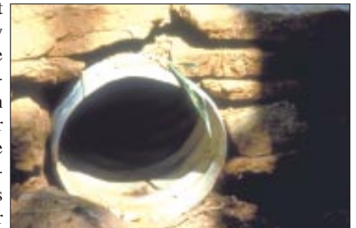
Culverts are commonly used in road construction.
